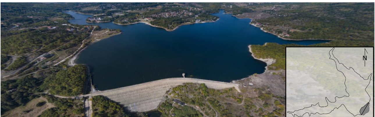
Figure 2. Aerial view and top-down footprint of the Dam and lake on the Brestovačka river (source: www.google.maps.org ).
